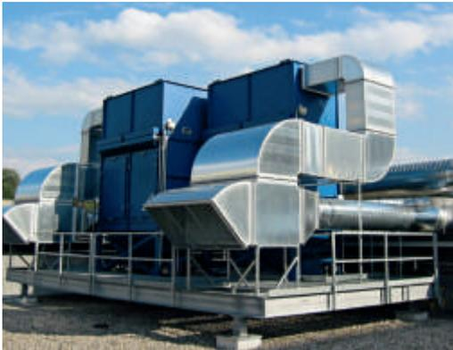
Dust-collection system with a thermal surface-finishing system, with heat recovery, and with air-volume of 2 x 15,000 Bm<sup>3</sup>/h.
