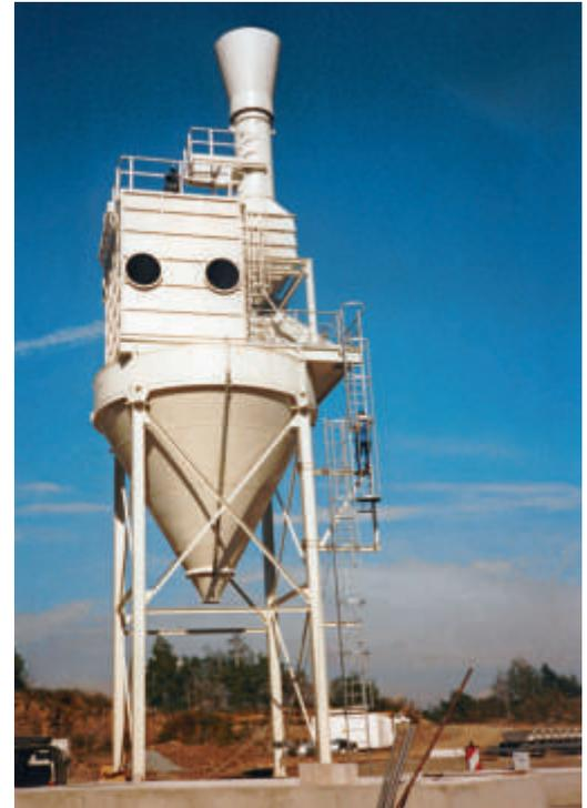
Air-suction exhaust for a crusher system, in a limestone plant.
