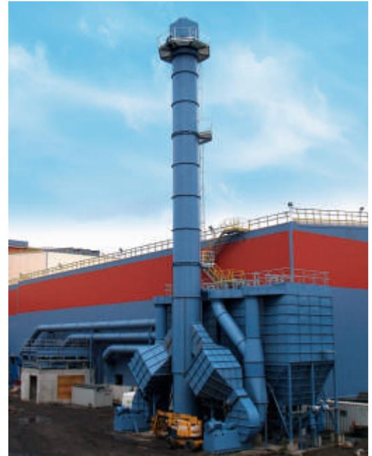
Hot-slab-ingot grinding system in Belgium, with volume flow of 300,00 Bm<sup>3</sup>/h.
