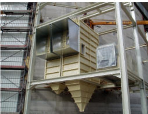
Climate control of a 50,000-metric-tonne sugar silo with dust-collection system, for the conveyor sections, during the installation phase.
