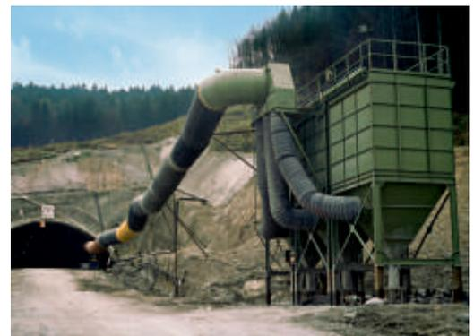
Dust collection in tunnel construction, for better working conditions.
