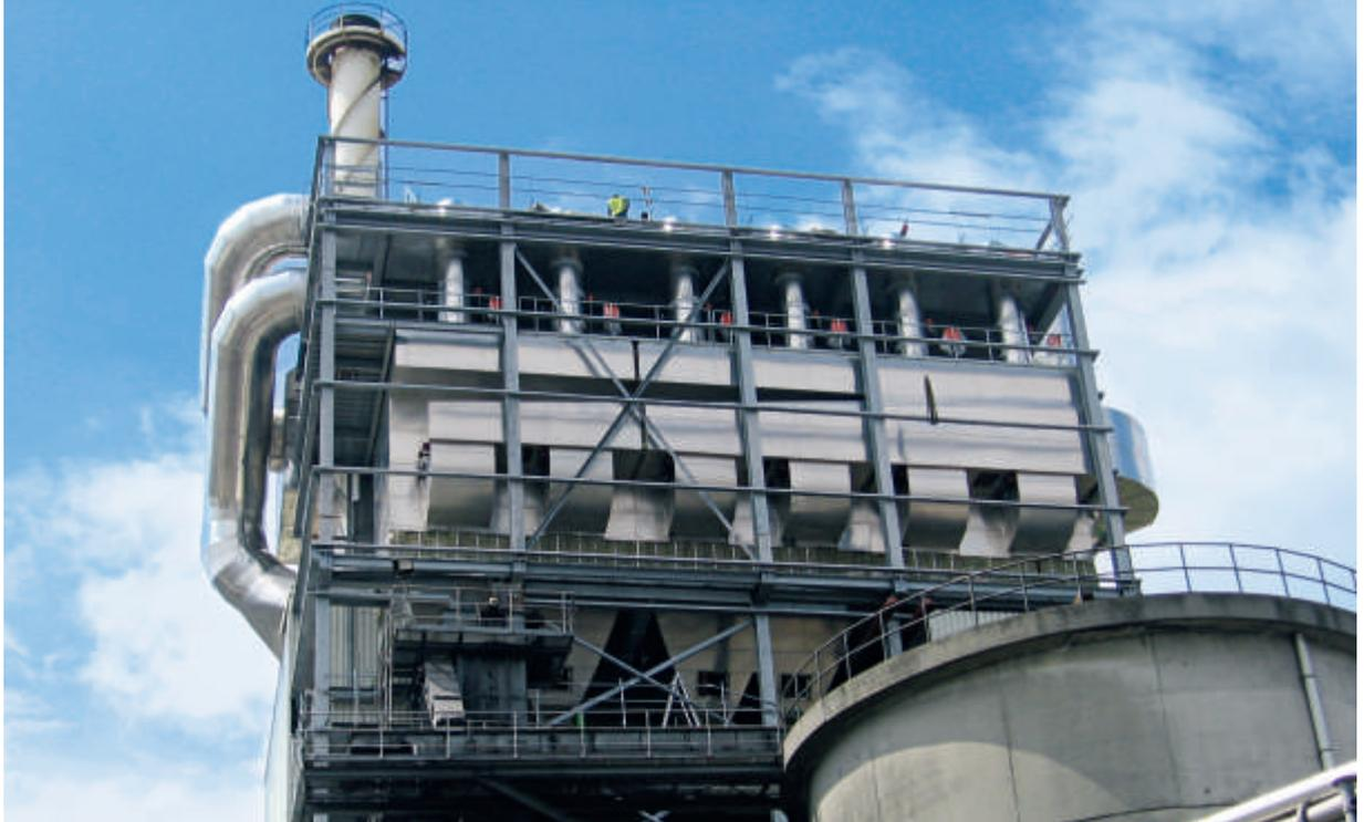
Flue-gas cleaning from coal-fired facilities, with residual-material combustion, including additive provision and disposal of airborne dust, is one of our specialties. Total air volume: 165,000 m<sup>3</sup> at 160°C operating temperature
